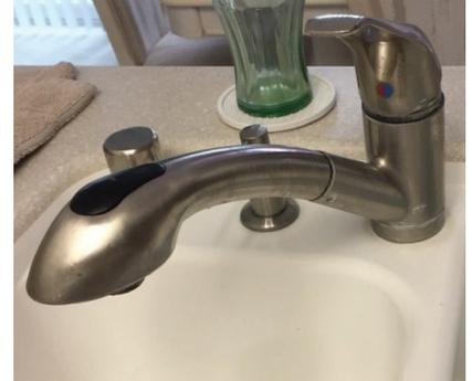
This faucet was leaching large amounts of lead into drinking water. With LeadSmart, the problem was easily detected and once the faucet was replaced, lead levels were reduced to compliant levels.
